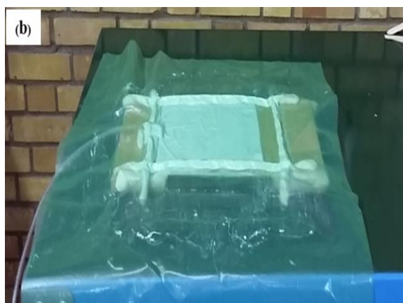
Fig. 4 The manufacturing steps of specimens: a) laying-up of lower composite layer on the flat mold and placing the flat mold under the fixture and HGFs b) vacuum bagging of laminate
