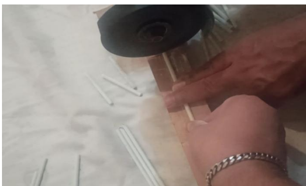
Fig. 4 Cutting GFRP reinforcing rods
