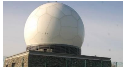
Fig. 1 composite radome for Meteorological radar
