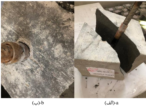
Fig. 10 (a) Cracking and splitting path of UHPC specimen without fibers (b) Splitting failure for UHPC specimen with 2% of fibers by volume
